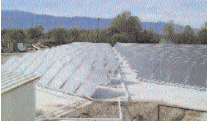
ABOVE Parking service Castellbisbal SA, container washing, Barcelona, Spain. Installed capacity: 357 kW th AIGUASOL ENGINEERING
